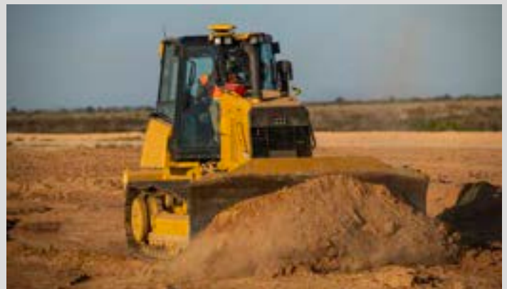
SITE PREPARATION – COARSE GRADING
